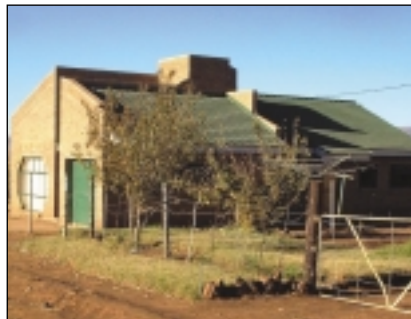
The house of Ms Sophie Nyalunga, a sales representative for Avroy Shlain and husband, Steven, who works as a data clerk. The couple stockpiled material and in total borrowed R22 000 to add six rooms to their small house
